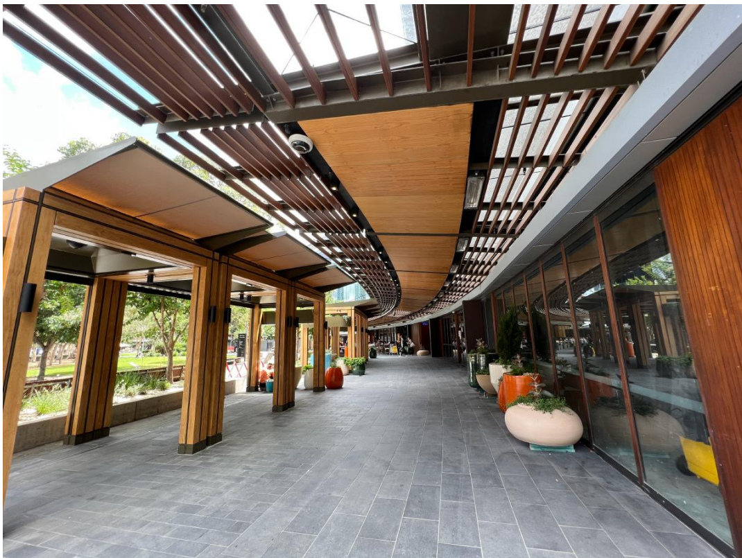
Figure 10: Retail terrace secondary pedestrian link, parallel to the pedestrian boulevard west of existing landscape planters and pergolas (proposed western outdoor seating area)
